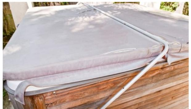
2. The Styrofoam cores inside the “skin” are wrapped in a sheet of plastic and then sealed. Over time the hot and cold weather causes the plastic inside to expand and contract until it finally breaks into small pieces. This allows rain water from the top, or steam from the bottom, to be absorbed into the cores. You’ll know this is happening when the cover slowly gets heavy and difficult to open. When you don’t want to use your spa because the cover is too heavy, it’s time to replace the cover.
