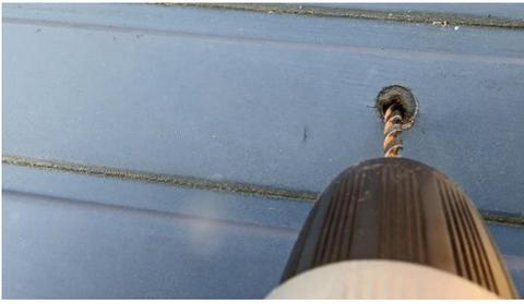
**Step 3.** Lay the old door on the new one and use the existing screw holes as a guide to drill new ones. Start with a ¼" drill bit, but don't be surprised if you have to make them larger when the time comes to install the door.
